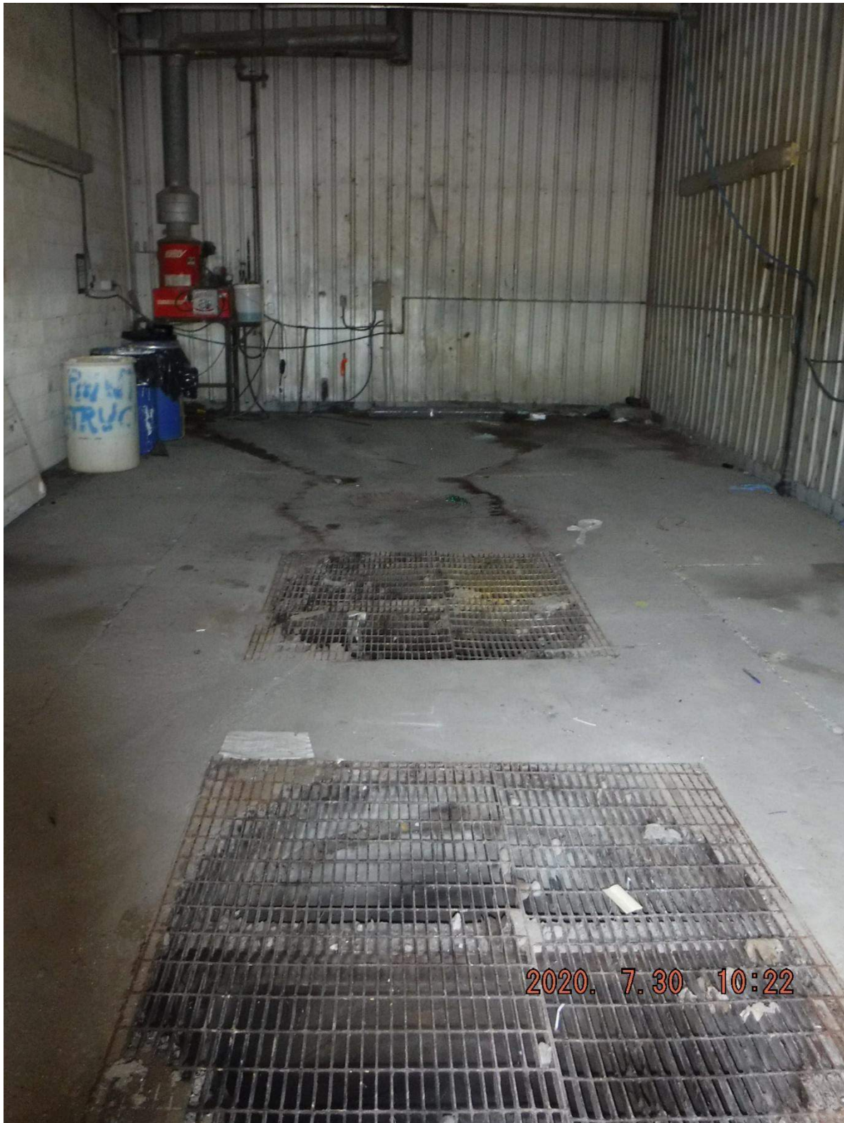
Photograph 5: Sumps located in the eastern wash bay former COL Public Works Shop
